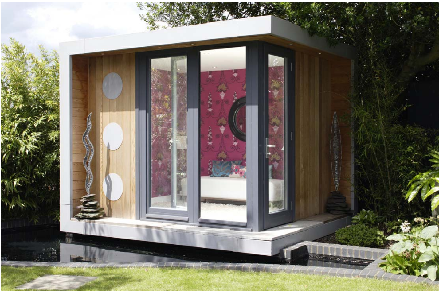
St.Albans, Hertfordshire - Constructed May 2007
